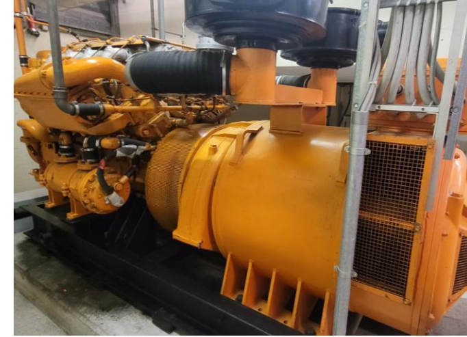
Notstromaggregat
